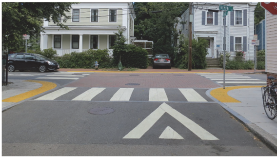
Raised Intersection in Cambridge, MA.
