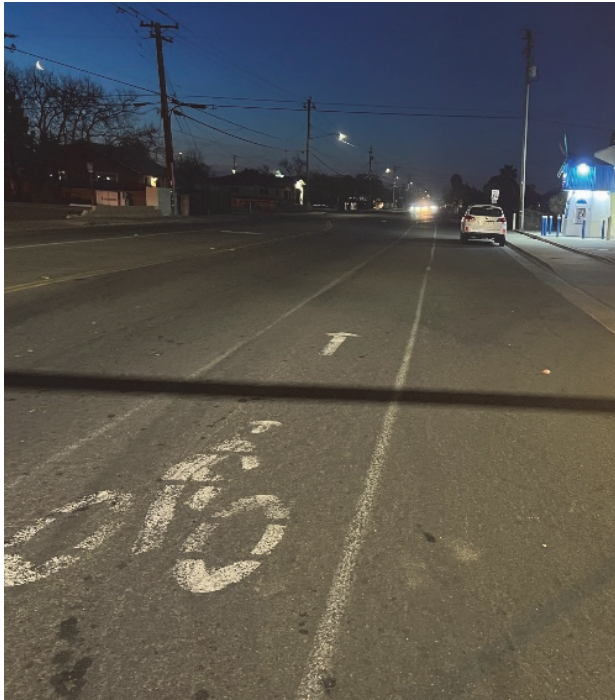
Class II Bicycle Lane on B Street passing OK's Food and Liquor south of Eighth Street.
