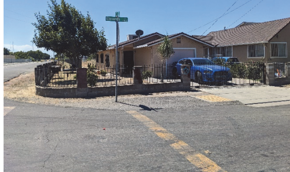
D Street and Eleventh Street crosswalk. Missing sidewalk and curb ramp.
