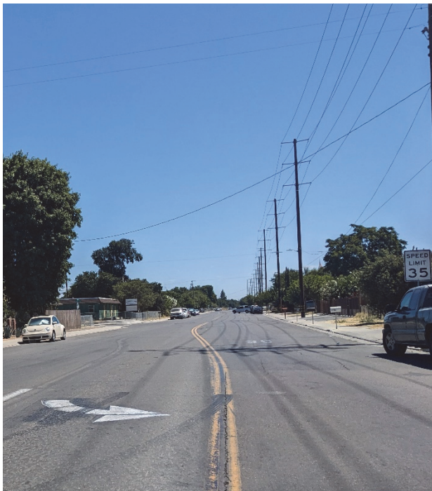
Lack of Bicycle Lanes and wide cross-section on Eighth Street.
